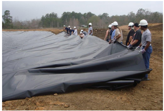
ArmorLiner panels easily deployed
