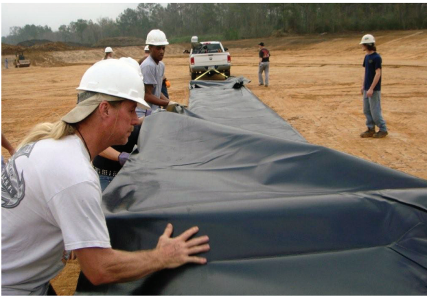
Fabricated panels being unrolled
