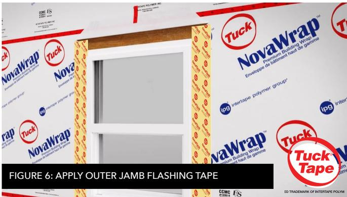
FIGURE 6: APPLY OUTER JAMB FLASHING TAPE
