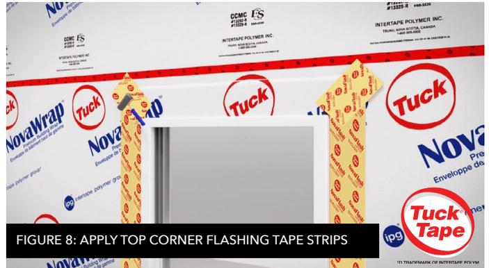
FIGURE 8: APPLY TOP CORNER FLASHING TAPE STRIPS
