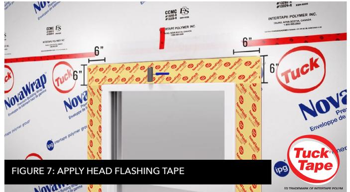
FIGURE 7: APPLY HEAD FLASHING TAPE
